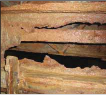
Photos 3 – 4: Typical environmental conditions in a shaft, which become more corrosive the deeper ones descends.
