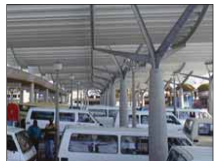
The "upside down spiders" on site following delivery. Notice the similarly grey tones of coating repair by "Zincfix".
