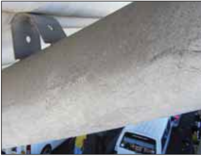
The curved hot dip galvanized tubular purlins are in excellent condition with a residual hot dip galvanized coating thickness of 134µm.
