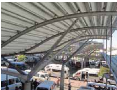
The connection pipe from one roof to the next was for some reason only painted, see condition left, which will in a short period of time have to be re-coated or replaced.
