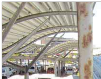
The connection pipe from one roof to the next was for some reason only painted, see condition left, which will in a short period of time have to be re-coated or replaced.
