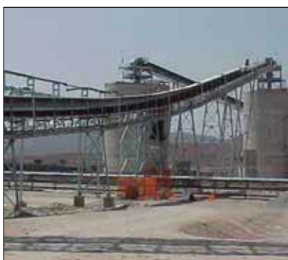
Photos 17 – 20: A number of views of Marula Platinum Smelter and the hot dip galvanized structural steel, including conveyor steelwork from an inclined shaft to varying process plants at the mine.
