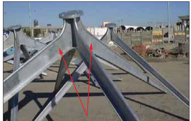
The "upside down spiders" on site following delivery. Notice the similarly grey tones of coating repair by "Zincfix".
