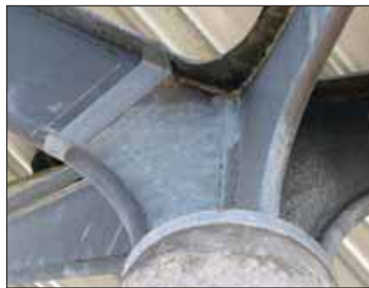
Where Zincfix has been correctly applied there are no signs of premature failure.
