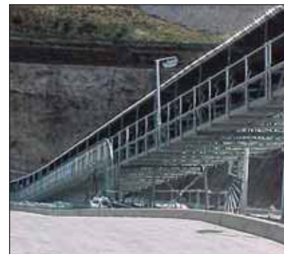
Photos 15 – 16: Early photos of the 6 500 tons of superstructure hot dip galvanized steel at Bafokeng-Rasimone Platinum Concentrator Plant.
