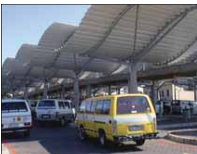
Varying views of the transport interchange upgrade showing the curved tubular purlins.
