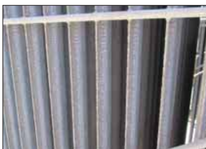
Edge of the radiator (above left) and close up of the edge of the radiator showing visible marine chloride salts and an area cleaned for taking coating thickness readings (above right).
