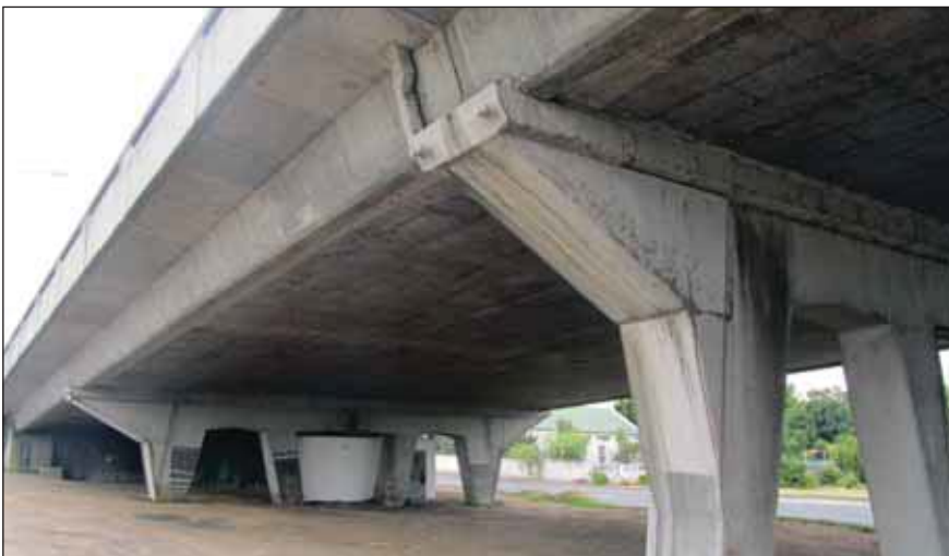
The above photos show the duplex coated steel corbel which while slightly discolored from rain water remains successfully intact.
