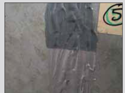
Photo 8: After exposure there was no physical deterioration of the Galvpatch repair material.
