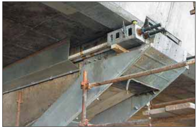
Positive anchoring of widened pier elements to the existing by using GEWI post tensioned anchors.
