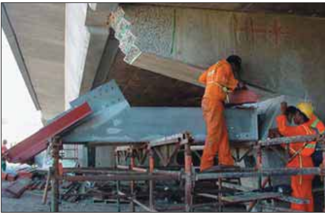
Preparation of the existing reinforced concrete pier to accommodate the hot dip galvanized structural steel corbel and strut.
