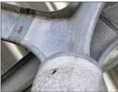
Due to the application thinness of Zincfix (achievable by thinly spreading the product with one's finger) the welded area is showing signs of premature corrosion.
