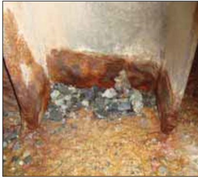
Photos 3 – 4: Typical environmental conditions in a shaft, which become more corrosive the deeper ones descends.
