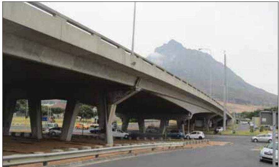
The Liesbeeck Parkway intersection looking towards Table Mountain showing the duplex coated steel corbels.
