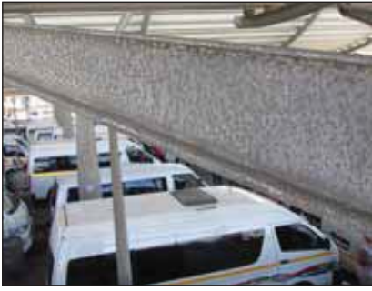
The "upside down spiders" showing atmospheric surface contamination.
