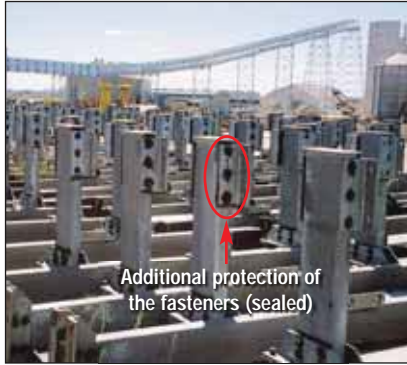
The shaft provides continual access for men, materials, machinery and ore, maintenance free performance of upwards of 25 years and is required to minimise routine downtime allowances. Photos 5 and 6 show hot dip galvanized shaft guides (left) and buntons and connections (right). Note the additional paint coating at crevices and over the fasteners.
