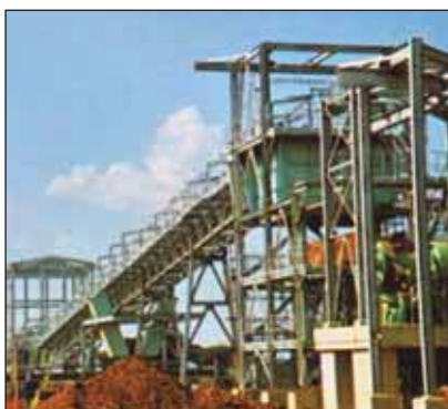
Photos 15 – 16: Early photos of the 6 500 tons of superstructure hot dip galvanized steel at Bafokeng-Rasimone Platinum Concentrator Plant.
