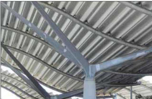
Some silver zinc rich spray paint was used, which is irritatingly highlighted against the stable hot dip galvanized zinc carbonate patina.
