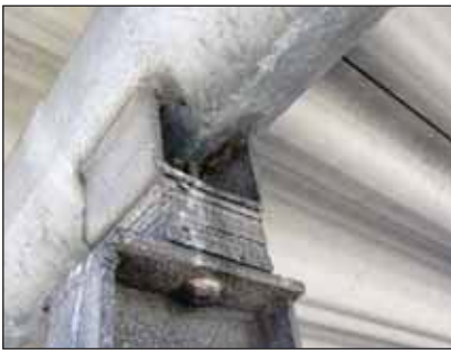
Hot dip galvanized I-Beam tubular purlin support, showing a residual coating thickness of 252µm.
