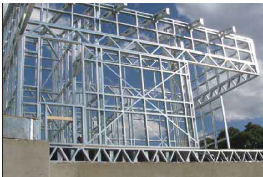
LSF structure of the renovation project that was broadcasted on KykNet. The 2nd floor was completed in 46 days.
