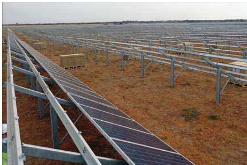
Solar panels being attached to installed galvanized steel structures.
