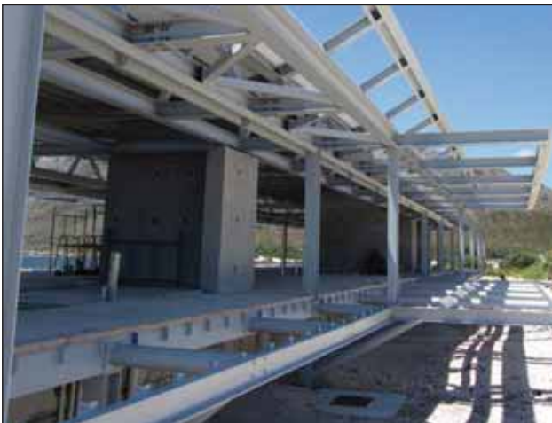
A view on the back side of the structure before cladding.
