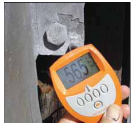
Damage which has occurred to a thick brittle coating that was not blasted prior to hot dip galvanizing.
