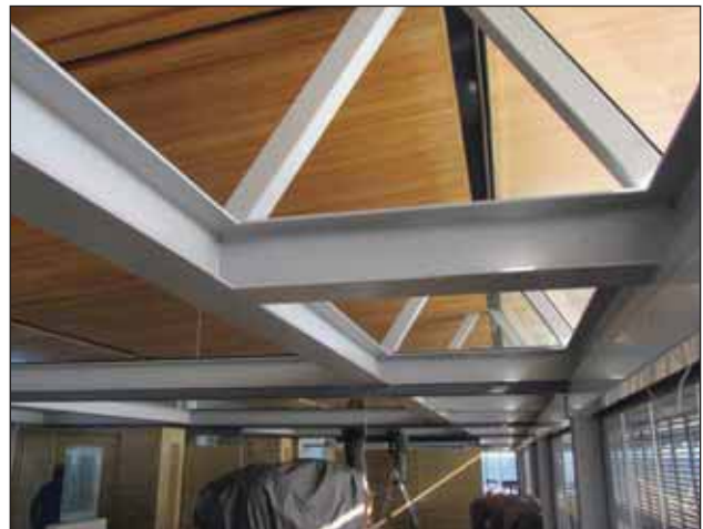
Inside the house showing the extent of the structural steel required to resist the load of the hydraulically operated patio doors.
