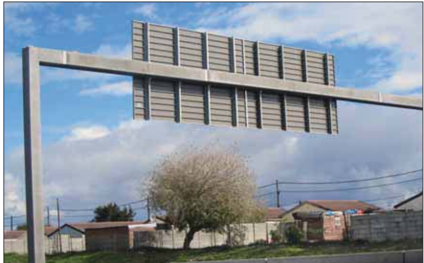
General view of the sign gantry.
