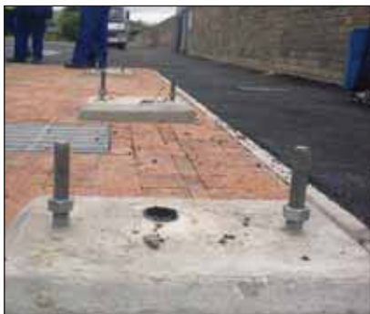
Photo showing the cast in hot dip galvanized anchor bolts and over sized nuts ready to accommodate a bus shelter:
