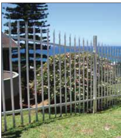
A no maintenance hot dip galvanized palisade fence will work in the majority of the environments in SA.
