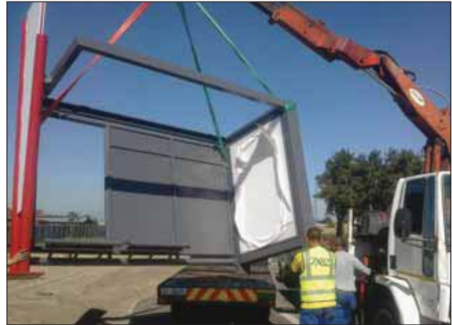
Lifting one of the finished bus shelters to its final position on site.
