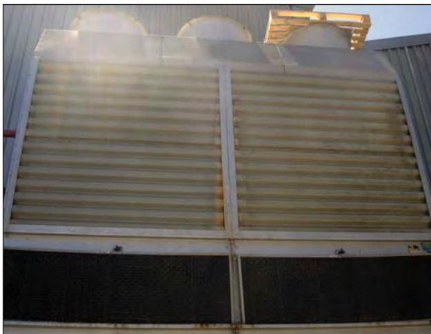
Photo 1: The 4-year old air condenser (A).
