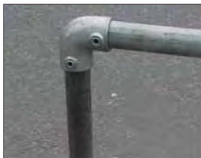
Specialised sockets eliminate or minimise the need for coating repair.
