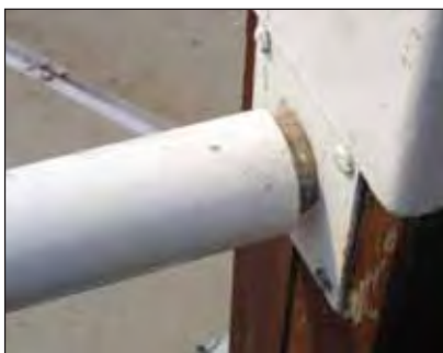
Sliding and specialised joints eliminate or minimise the need for coating repairs.
