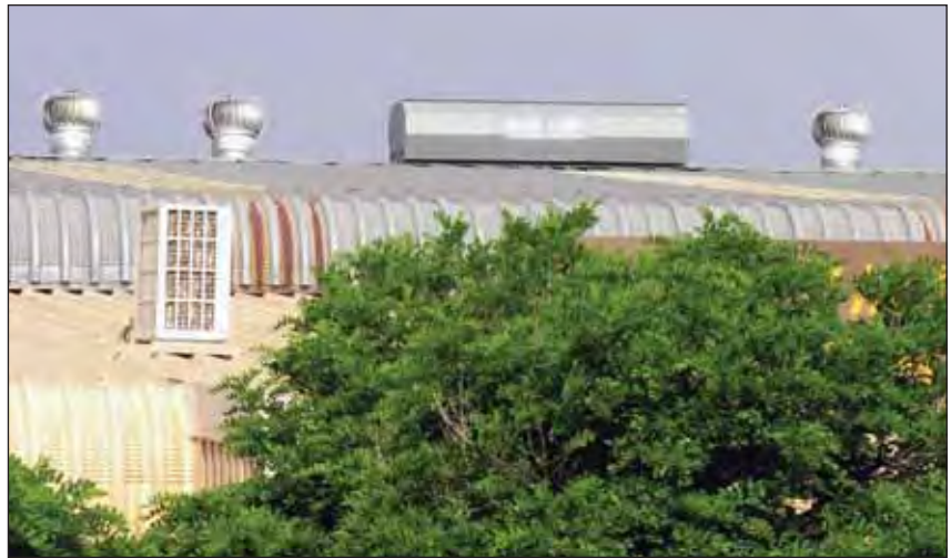
Photo shows discoloration of the galvanized sheeting immediately below the polymer roof sheeting.
