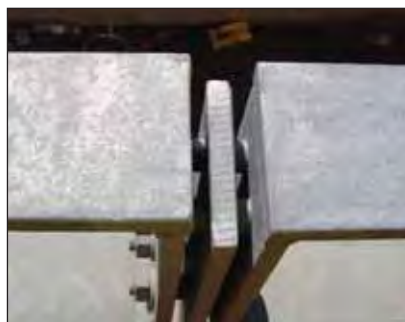
Sliding and specialised joints eliminate or minimise the need for coating repairs.
