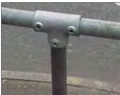
Specialised sockets eliminate or minimise the need for coating repair.
