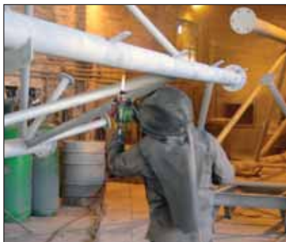
Photos 3 (left) and 4 (right) show the degree of difficulty in ensuring a uniform spread of zinc metal spraying to the specified coating thickness.
