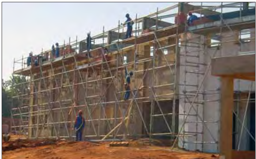
The hot dip galvanized scaffolding will be monitored for its service life durability.
