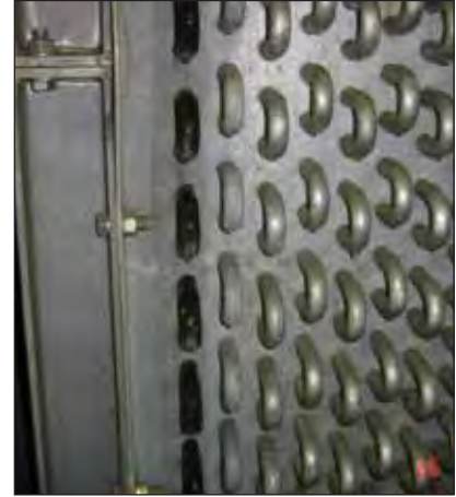
Little evidence of corrosion on the coil end of the operational installation.
