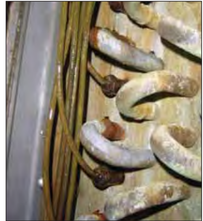
Severe corrosion is taking place on every second pipe of the coil at both coil ends where copper pipes are attached.
