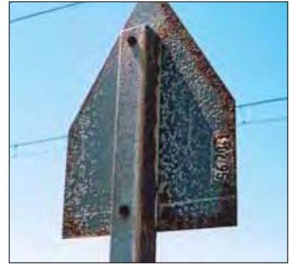
One side of pole the hot dip galvanizing is totally corroded due to a combination of sea salt, moisture and lack of drying from the sun.
