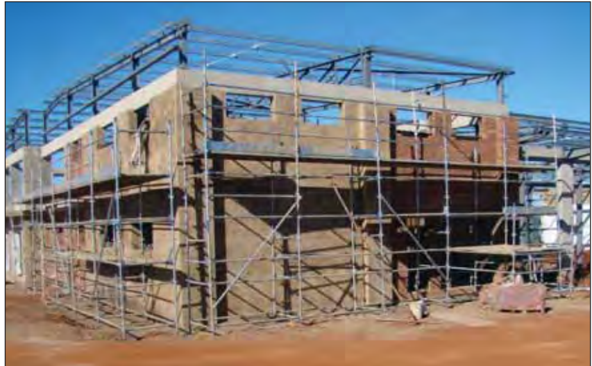
Other than being cleaned of cement deposits, which do not affect the life of the coating, the hot dip galvanized scaffolding can be easily monitored for its performance over its service life.
