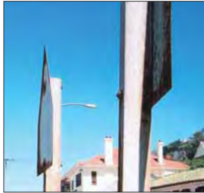
One side of the sign post, due to the full sun has no corrosion.
