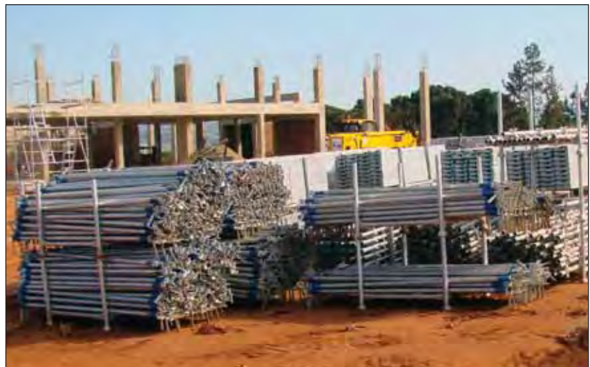
Hot dip galvanized scaffolding stacked on site for imminent erection.
