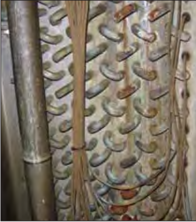
Corrosion evident on the coil end of the non-operational coil.
