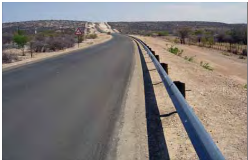
Photos 1 and 2 above show the installed and about to be installed guardrails on the road from Kamanjab to Omagange, Namibia.
