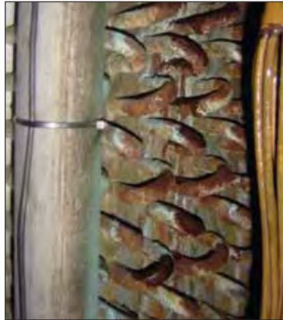
Severe corrosion is taking place on every second pipe of the coil at both coil ends where copper pipes are attached.
