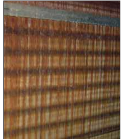
Corrosion evident on the coil fins on the inside face of the bread cooling chamber. Note the corrosion evident on every second pipe within the heat exchanger, with corrosion of the fin in contact with the corroding pipe.
