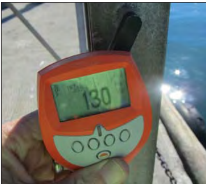
Zinc chloride salts removed and the residual coating thickness measured - 130µm.
