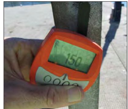
Zinc chloride salts removed and the residual coating thickness measured - 150µm.
