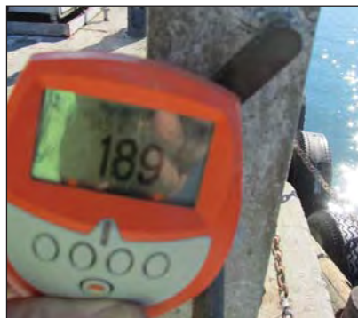
Zinc chloride salts removed and the residual coating thickness measured - 189µm.
