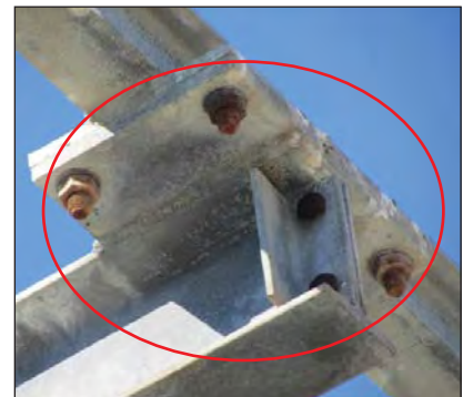
Photos above show the gantry with some uncoated carbon steel that has been added. This will in time tend to discolour the hot dip galvanizing when the former begins to rust. Photo right shows the inappropriately coated fasteners, which were most probably originally only zinc electroplated, requiring replacement or coating repair.
