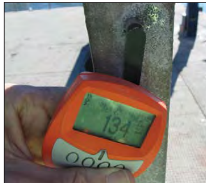
Zinc chloride salts removed and the residual coating thickness measured - 134µm.
