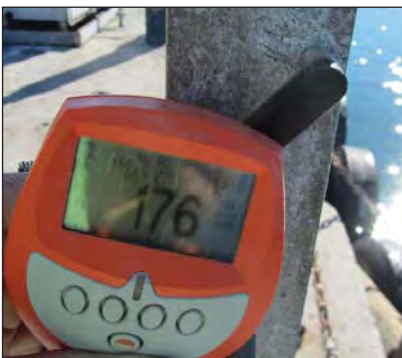
Zinc chloride salts removed and the residual coating thickness measured - 176µm.
