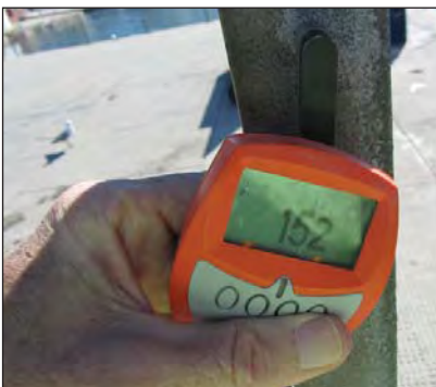
Zinc chloride salts removed and the residual coating thickness measured - 152µm.
