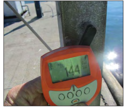
Zinc chloride salts removed and the residual coating thickness measured - 144µm.
