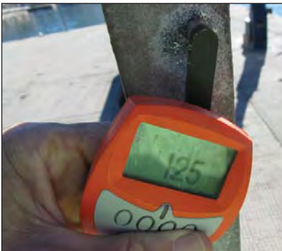
Zinc chloride salts removed and the residual coating thickness measured - 125µm.
