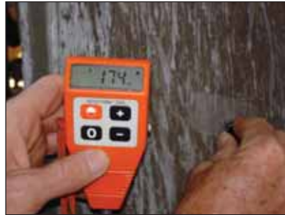
Coating thickness on structural steel adjacent to the reagent area.
