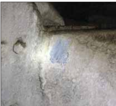
The hot dip galvanized coating thickness on station steelwork proved to be in good condition.
