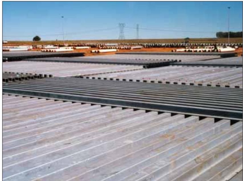
Hot dip galvanized shaft guides correctly laid out on site, awaiting installation in the shaft.
