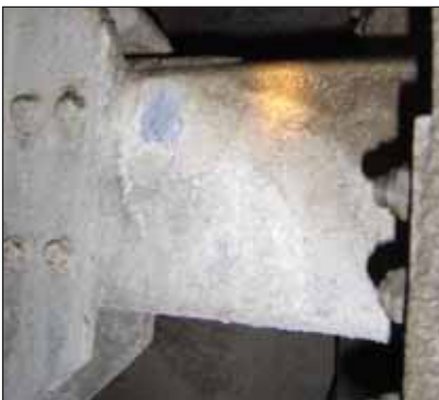
The coating thickness on shaft buntuns at four different levels were inspected but as they were similar in residual coating thickness, only two have been reported. The calcerous growth in most instances was removed prior to measuring the residual coating thickness.
