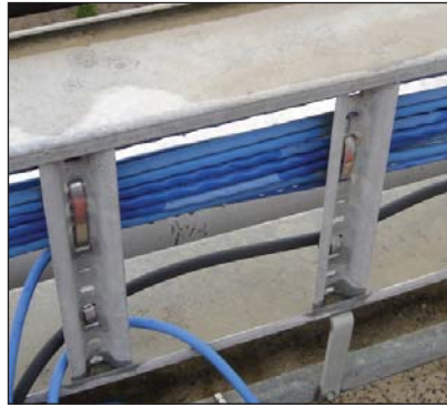
Photo left shows the A&S Cable ladder in the foreground and a more modern edge mounted cable ladder in the background. Centre shows a close up of the A&S Cable ladder and right, residual coating thickness on the cross rung (89.5µm).
