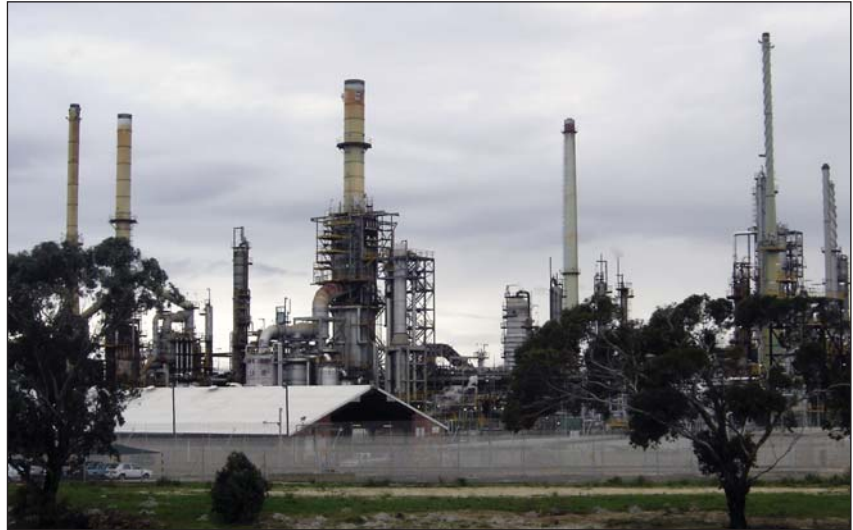
The general view on the petro chemical plant in Milnerton.
