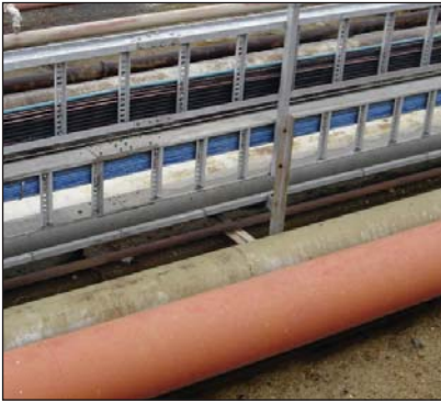
Photo left shows the A&S Cable ladder in the foreground and a more modern edge mounted cable ladder in the background. Centre shows a close up of the A&S Cable ladder and right, residual coating thickness on the cross rung (89.5µm).
