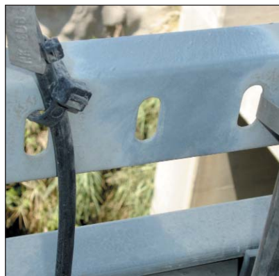
Cable ladder cross rung.
