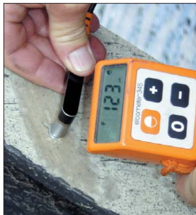
Hot dip galvanized coating thickness (paint removed).
