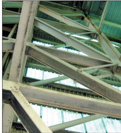
General photo of the structure.
