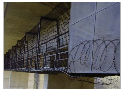
Left – A general view of the bridge from the landward side (the bungi jumping ropes can be seen in the centre of the bridge) and right - a view of the access walkway looking from the east end, fixed to the underside the bridge on the seaward side.
