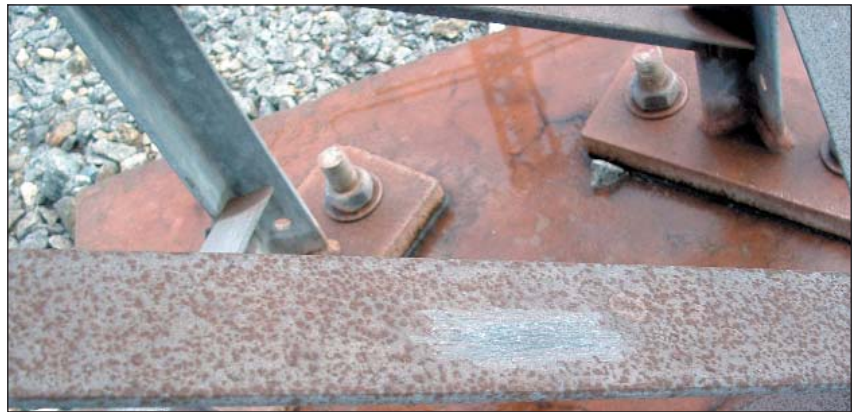
Despite the apparent "rust" contamination of the galvanized surface, once removed the galvanized coating measured 126µm.
