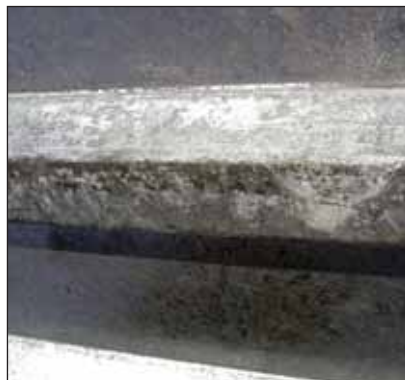
Deposits of wet storage stain have been removed from the sheeting.
