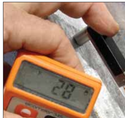
Coating thickness readings have been taken and are still above the requirements for a Z275 class of coating.
