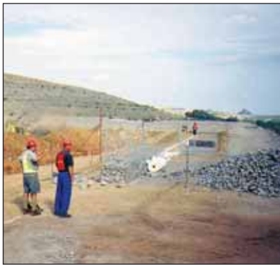
Starting Terramesh™ installation.
