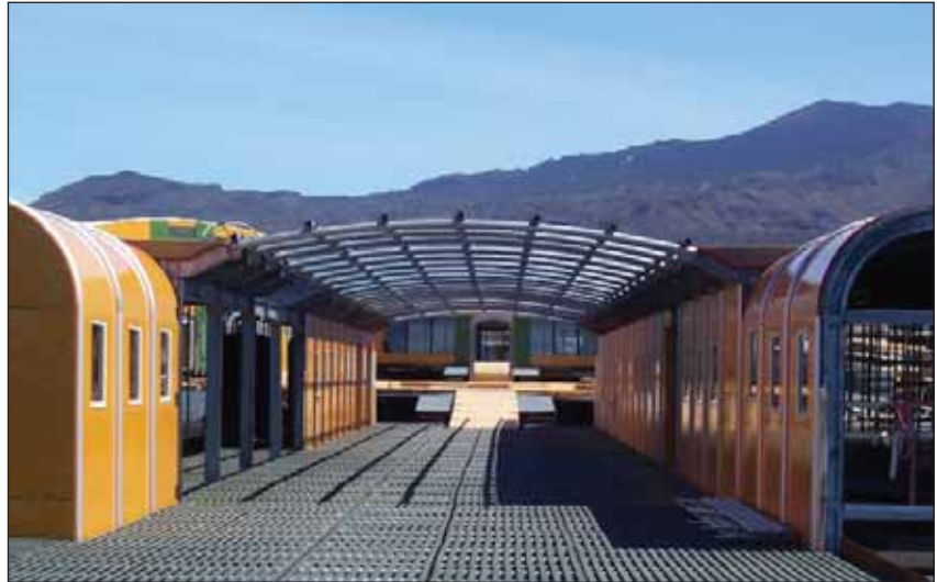
Mentis Positive Non-Slip Hot Dip Galvanized Grating was used on all the walkway areas between the harbour and the station.
