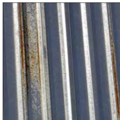
Close up of the side sheeting.
