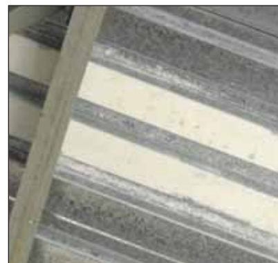
Thoroughly clean all heavily white rusted areas on the undersides of the sheeting of the building prior to any subsequent coating repair.
