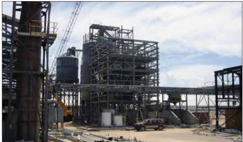
General view of part of the "dry plant" under construction, which will ultimately be used in the refining of titanium products.
