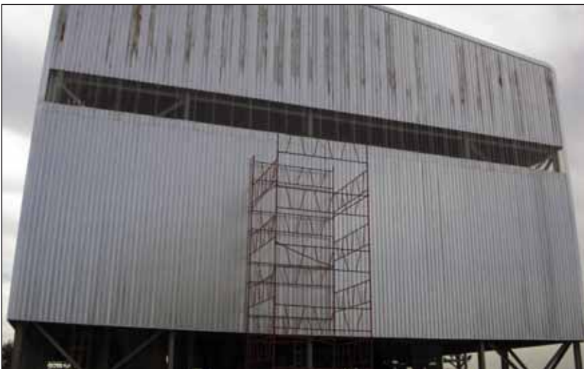
General view of the end sheeting.
