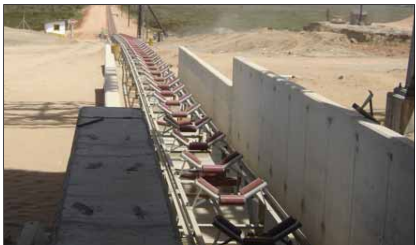
The starting point of the 4km overland hot dip galvanized conveyor that ends at the sea pier from where refined products will be loaded onto sea-barges.
