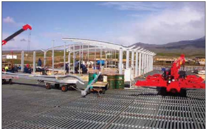
Andrew Mentis Positive Non-Slip Hot Dip Galvanized Grating is the solution for the Weather Base Station on Marion Island.
