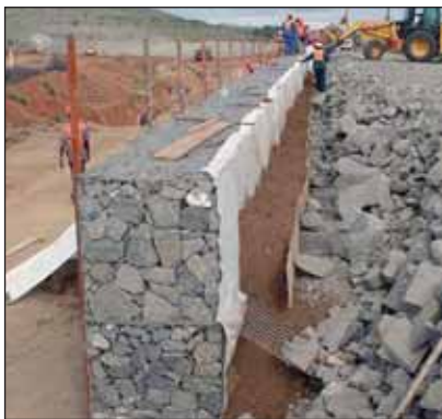
Starting the continuous hot dip galvanized wire Terramesh™ installation.
