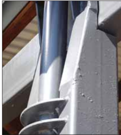
Some protuberances and general coating roughness, normally acceptable when only hot dip galvanizing is required, should be removed prior to painting – see HDGASA 03-2006.
