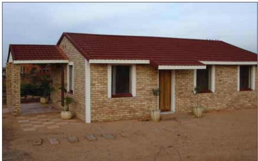
Newly constructed light steel frame single story building clad with brickwork.
