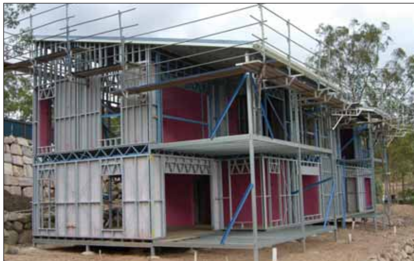
Double story light steel frame building during construction.
