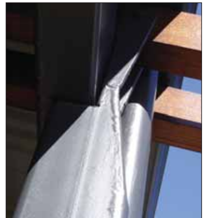
Photos above show unacceptable coating roughness and a zinc run at the weld area, which should ideally have been removed prior to painting.
