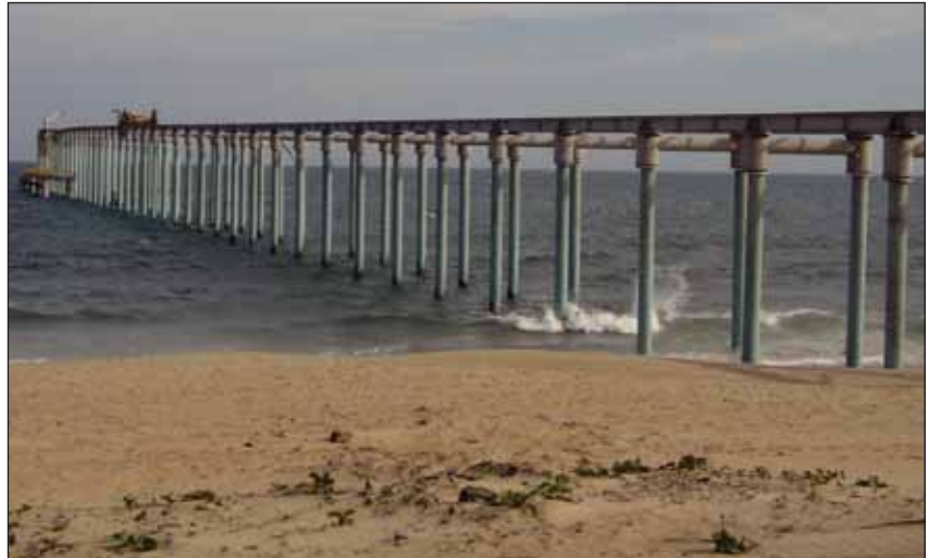
The sea pier and conveyor termination from where refined product will load onto sea-barges for trans-shipment to ships anchored off shore.
