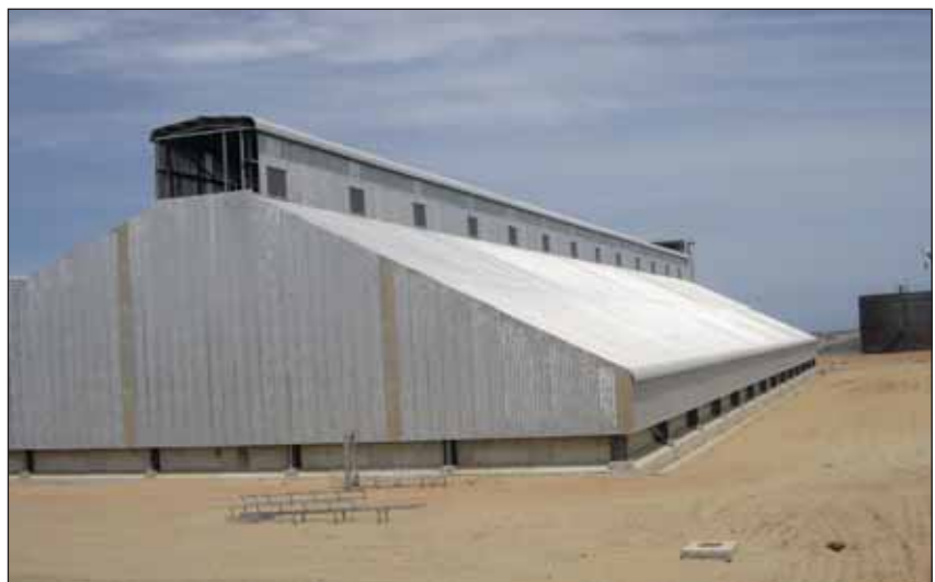
One of three such structures, where refined products will be stored prior to conveyance, via an overland conveyor, to a specially constructed loading pier, for loading onto sea-barges for transhipment to ships anchored offshore
