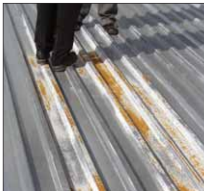
General view of the roof sheeting showing deposits of wet storage stain and subsequent red rust.
