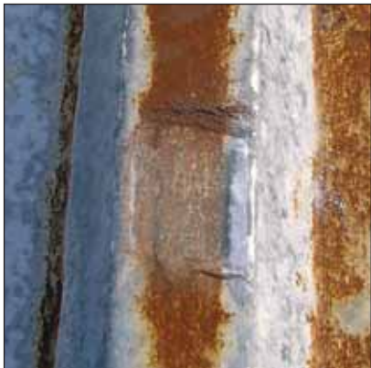
Red discoloration has been removed.
