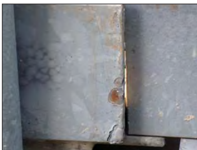
Damaged coating in reagent loading area.
