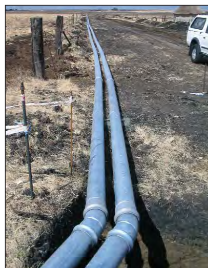
When Lula is installed above ground the system cannot be tampered with as there are no couplings to remove.
