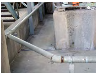
Hot dip galvanized water pipe in the reagent area.
