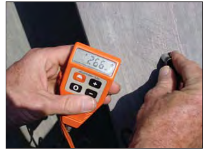
Coating thickness on structural steelwork in the wet screening area.
