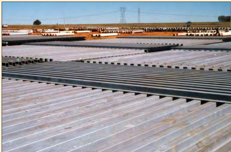
Hot dip galvanized shaft guides correctly laid out on site, awaiting installation in the shaft.
