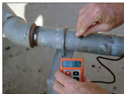
Coating thickness of a hot dip galvanized water pipe in the reagent area.
