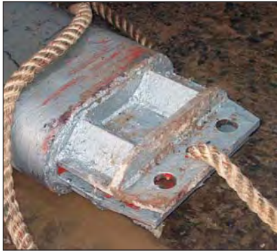
A close-up photo showing the new buntion bracket welded to the buntion, ready for slinging down the shaft.
