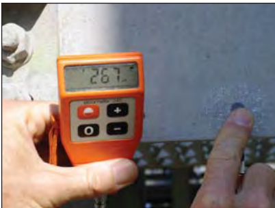
Coating thickness on the hot dip galvanized crusher conveyor steelwork.
