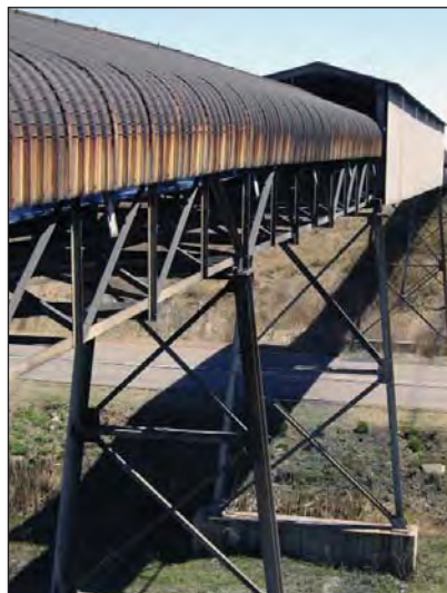
The hot dip galvanized structural steelwork supporting the overland conveyor at an access road, is still performing exceptionally well after 20 years of service.
