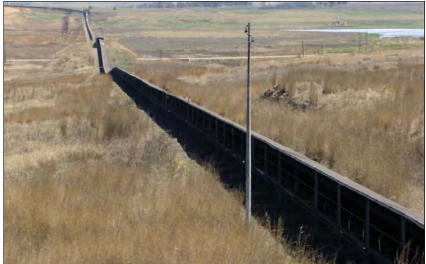
The V3 overland conveyor has been exposed to the elements for in excess of 20 years.
