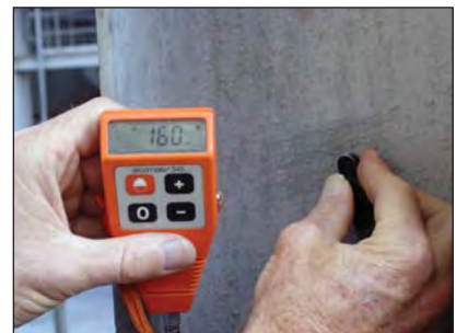
Coating thickness on structural steel in the floatation area.
