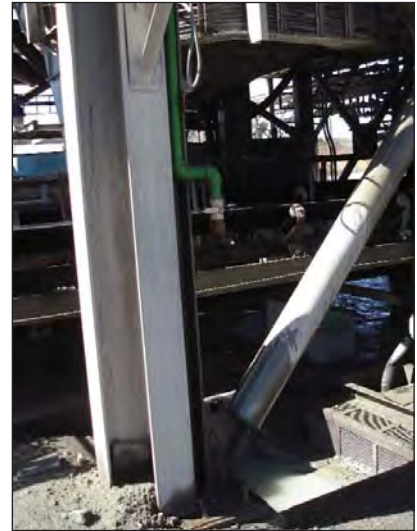
Hot dip galvanized structural steel in the wet screening area.
