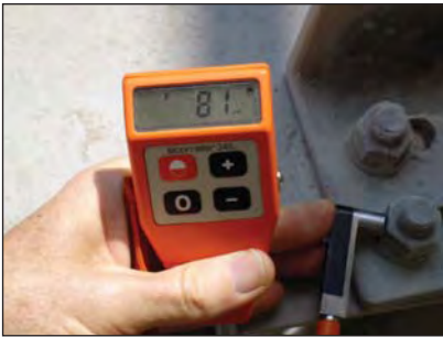
Coating thickness on the hot dip galvanized nuts on the crushing plant conveyor steelwork.
