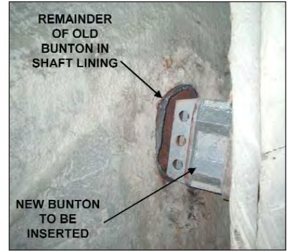
The buntion has now been cut off and the new buntion is ready to be installed
