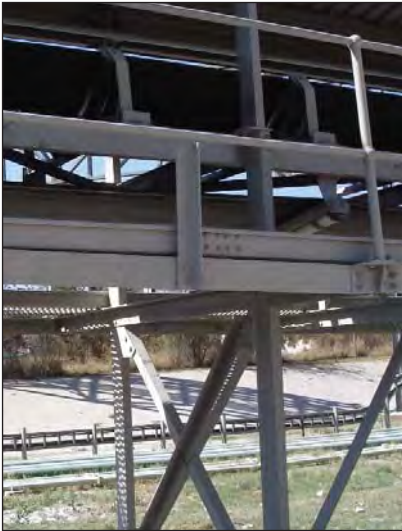
Hot dip galvanized structural steel supporting the crushing plant conveyor.
