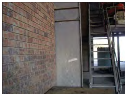
Hot dip galvanized structural steel in the floatation area.
