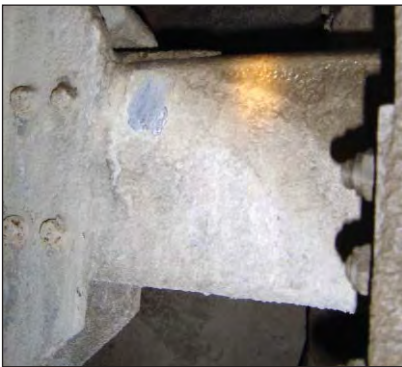
The coating thickness on shaft buntons at four different levels were inspected but as they were similar in residual coating thickness, only two have been reported. The calcerous growth in most instances was removed prior to measuring the residual coating thickness.
