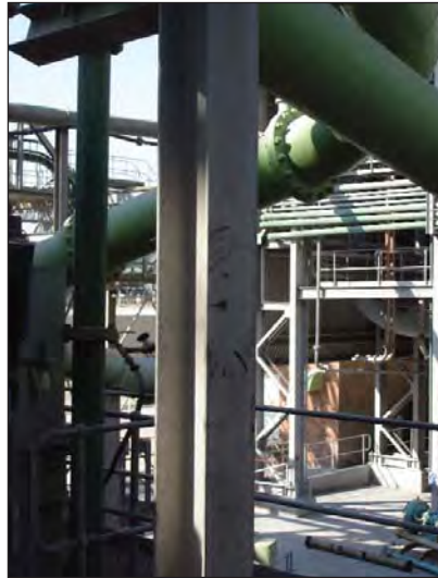
Hot dip galvanized structural steel in the milling area.
