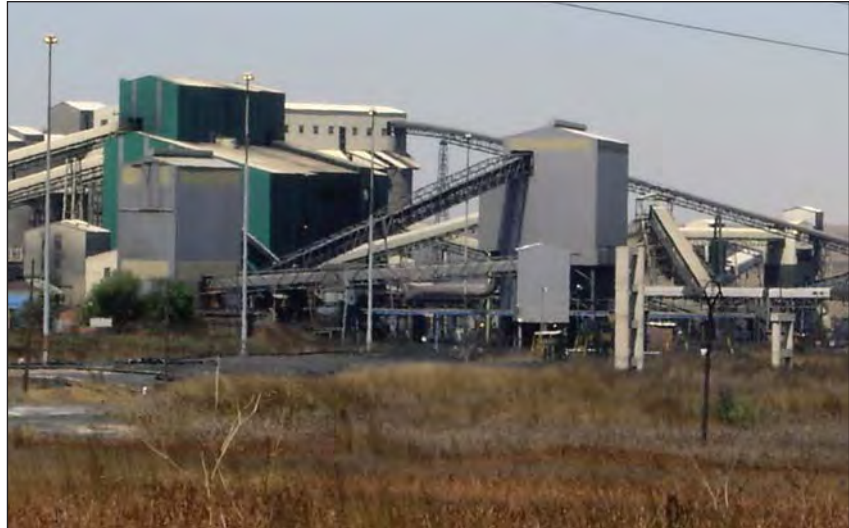
General view of Douglas Colliery.
