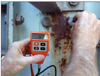
Photo 1: Comparison between hot dip galvanizing and paint in the reagent area.
