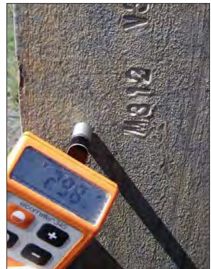
Coating thickness readings taken on the supporting structural steelwork at the access road were still in excess of that required by the specification.
