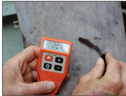
Coating thickness on structural steel in the milling area.
