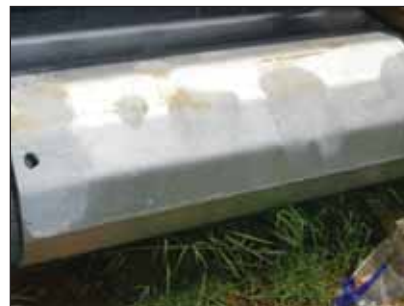
Photos 6, 7 and 8 (left to right). Taken of one particular mast where it is felt that excessive coating repairs have been undertaken.
