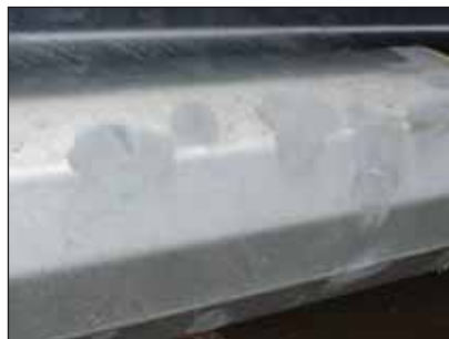
Photos 6, 7 and 8 (left to right). Taken of one particular mast where it is felt that excessive coating repairs have been undertaken.
