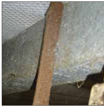
Hot dip galvanized purlin in the bulk tank room.
