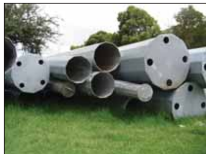
Photo 1. The stacking of the masts on site. The absence of timber dunnage required to prevent inappropriate component contact, when offloading and stacking, has lead to unnecessary coating damage.
