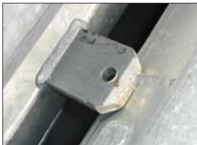
Photos 16, 17 18 and 19 (clockwise from top left) show how inappropriate stacking on site, particularly when weld on gusset plates and sharp corners clash, can cause coating damage.
