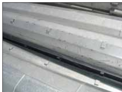
Photos 14 (left) and 15 (right) – scuff marks on the sides of some of the masts.
