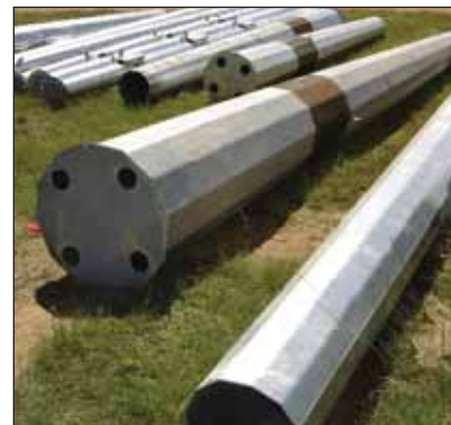
Photos 20 (left) and 21 (right) show revised stacking of the masts on site. Due to the abundance of lay down areas, this was seen to be more acceptable, however, coating damage had already occurred from previous offloading and incorrect stacking.
