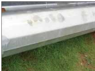
Photos 6, 7 and 8 (left to right). Taken of one particular mast where it is felt that excessive coating repairs have been undertaken.
