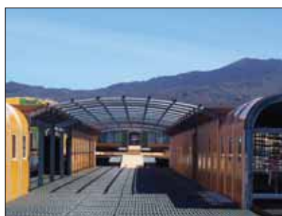
Various views showing the hot dip galvanized steel used in construction of the base.
