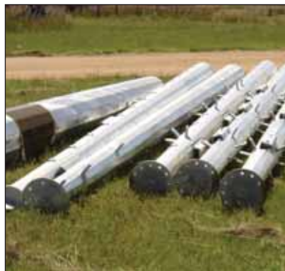
Photos 20 (left) and 21 (right) show revised stacking of the masts on site. Due to the abundance of lay down areas, this was seen to be more acceptable, however, coating damage had already occurred from previous offloading and incorrect stacking.
