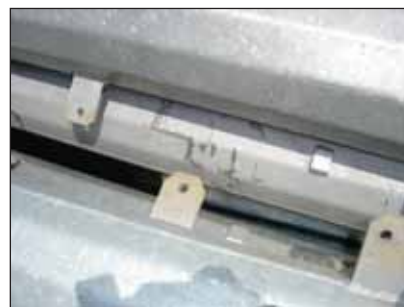
Photos 9, 10 and 11 (left to right). Mechanically damaged coatings due to inappropriate transportation, handling and stacking.
