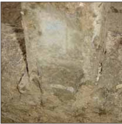
Base of cattle separation barrier post, showing the build up of cattle dung etc.
