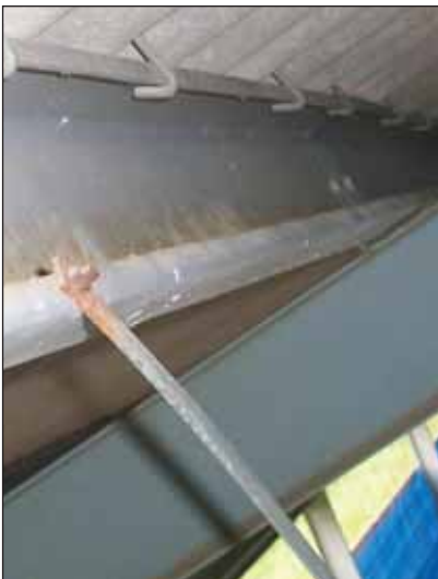
A combination of the acidic washdown chemical, wood chips and fairly humid environment has resulted in a poulitice on the inside of the lip channel, resulting in accerated corrosion.
