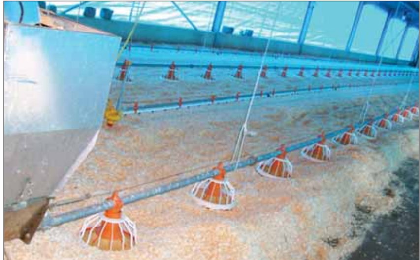
Inside the chicken house showing the wood shavings and feeding units, notice the hot dip galvanized water supply piping.
