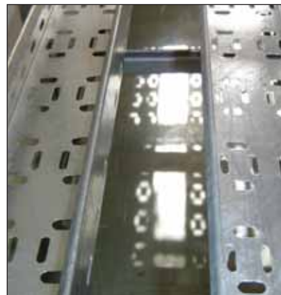
The cable tray on the right (hot dip galvanized to SANS 121) will out last the tray on the left (continuously hot dip galvanized material) by upwards of 4 times!
