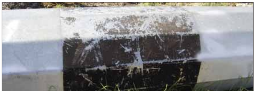
Photo 45 shows the paint coating that is added to this area of the masts to prevent differential aeration (necking corrosion) at the final soil/atmosphere interface. To prevent this type of corrosion in the long term, the paint coating needs to be reinstated.
