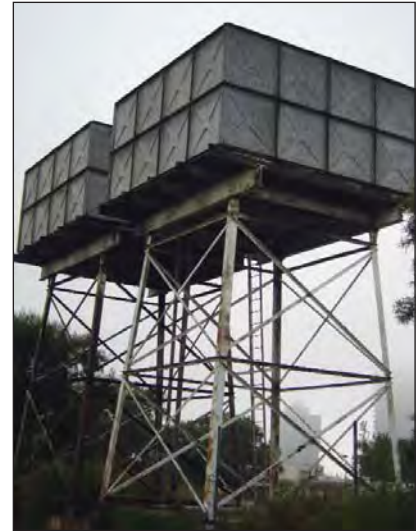
General view of water tanks.
