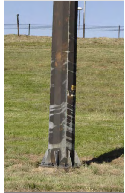
The general appearance of the matt grey and black weathered iron/zinc alloy hot dip galvanized coating.
