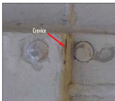
Figure 7: Crevice (potential corrosion area).
