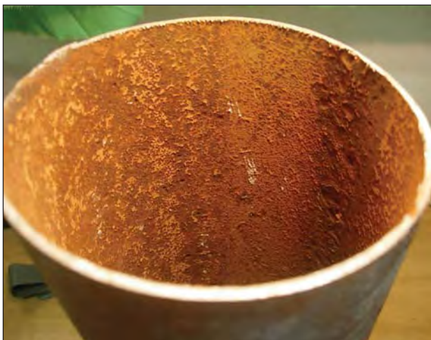
Figure 2: Corroded internal condition of the pipe section.
