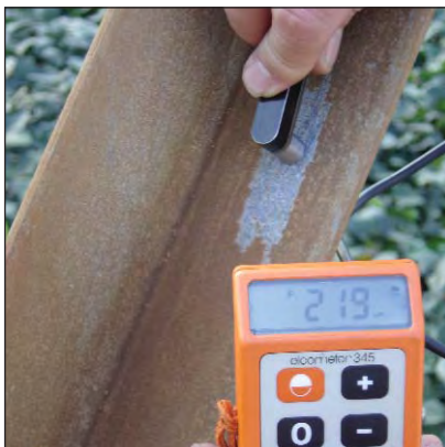
Coating 50 years old and still plenty of maintenance free life.
