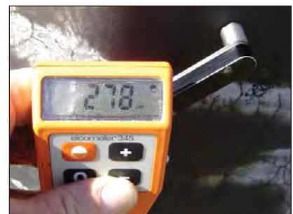
The matt black weathered coating thickness measured 278µm.
