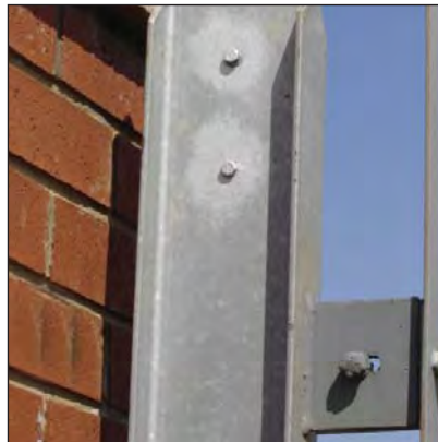
“Cold galv” encompasses many products, only some blend in with the final zinc patina, once formed.
