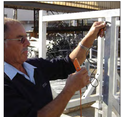
Coating inspection of the components is recommended at the galvanizer prior to delivery to site.
