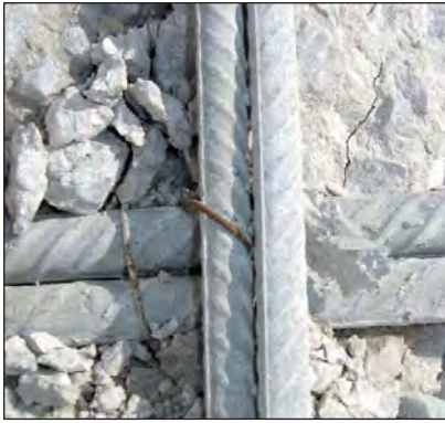
The condition of exposed hot dip galvanized reinforcement found during the demolition of the 40 year old bridge. With isolated exceptions, the hot dip galvanized reinforcing shown, in this photograph, is typical of 98% of that inspected.
