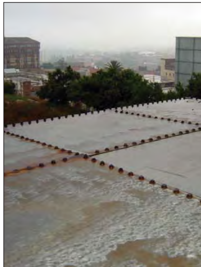
View on the roof looking north.
