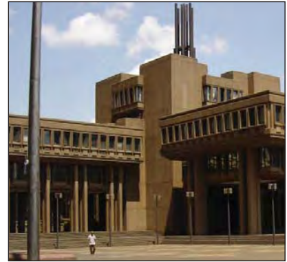
The slender pre-cast concrete panels that were used on the Civic Centre in Braamfontein were hot dip galvanized due to cover restrictions and to prevent spalling and rust staining. To date after some 30 odd years the panels are performing as expected.
