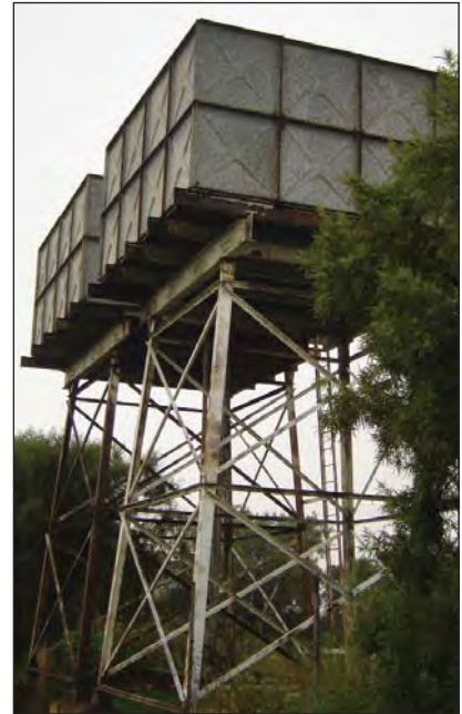
An old "Braithwaite" pressed steel tank (see Case History), supported by a painted steel structure.
