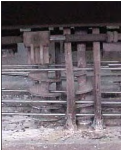
Pipes being immersed "screwed" into the molten zinc using a series of screw conveyors or augers. Immersion times are determined by the rotational speed of the augers.
