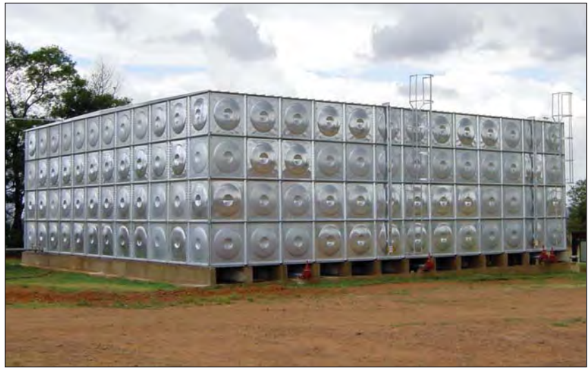
1 million litre pressed steel tank.
