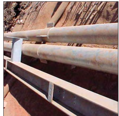
Wet trades are active adjacent to, and general site dirt may affect appearance of hot dip galvanized coating.
