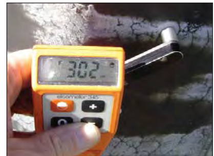
The matt grey weathered coating thickness measured 302µm.
