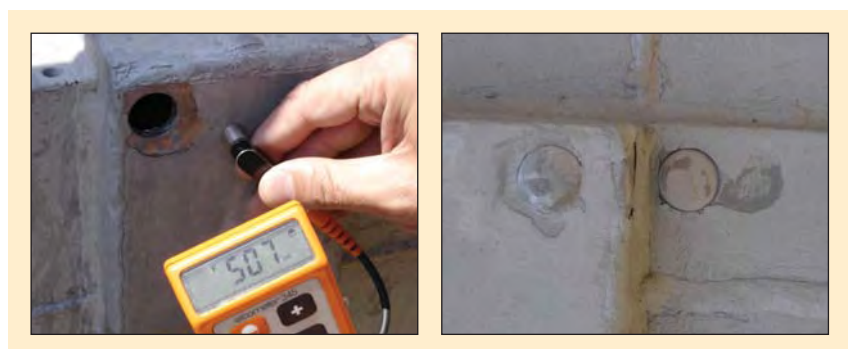
Figure 3: Mechanical damage caused by hammering steel plugs at most drainage holes.
