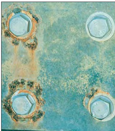
Figure 15. Stainless steel fasteners attached to hot dip galvanized plate in immersed conditions, note the sacrificial attack of the zinc coating surrounding uninsulated fasteners (in spite of the flat fibre washer the bolts still had electrical contact with the surrounding steel) compared with the insulated fastener (here the bolt fitted dead centre in the hole, resulting in no electrical contact) and consequently no attack of the surrounding zinc has taken place.
