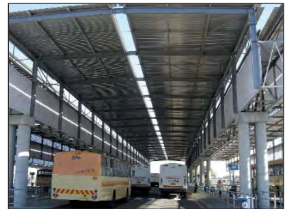
An end view of one of the bus shelters which forms part of the new Transport Interchange.
