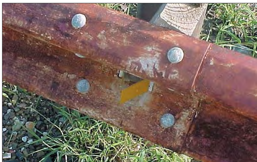
Hot dip galvanized bolts still providing corrosion protection.
