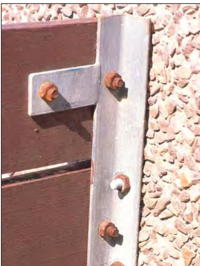
Figure 2. An assortment of zinc coated bolts showing the importance of coating thickness in a particular environment.
