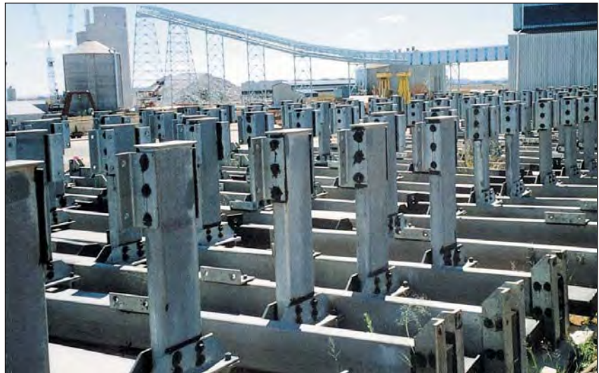
Hot dip galvanized shaft bunton sets providing horizontal supports for shaft steelwork in many mining operations have been assembled using hot dip galvanized lock bolt systems. In order to enhance the corrosion protection, all of the lock bolts were overcoated with a coaltar epoxy.
