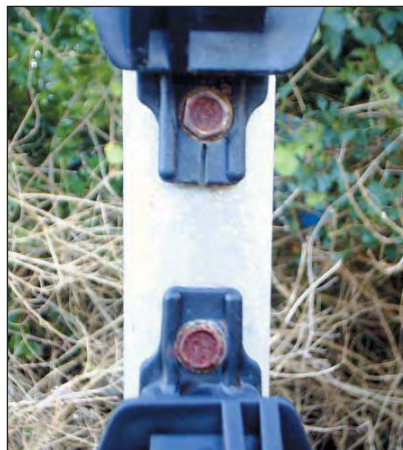
Electroplated screws used in less aggressive marine areas, surrounded by bush show corrosion after the same exposure time.
