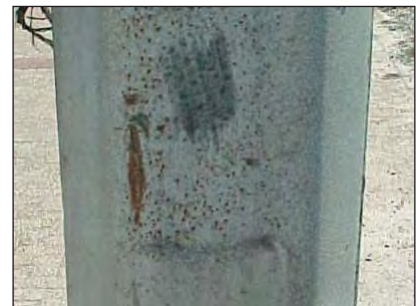
Close-up of the coating on the marine side showing the scraped surface.
