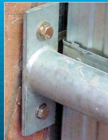
Electroplated expansion bolts offering less protection on steelwork projects that are hot dip galvanized for durability, no longer have to be tolerated by the specifiers.
