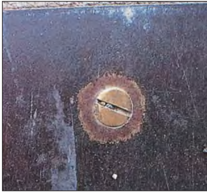
Figure 14. Brass bolt in hot dip galvanized steel on a parking deck.
