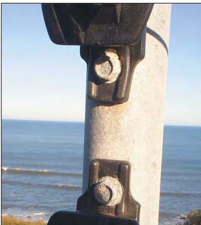
Hot dip galvanized self drilling screws installed at Westbank Golf Course show no corrosion after more than a year in a marine atmosphere.
