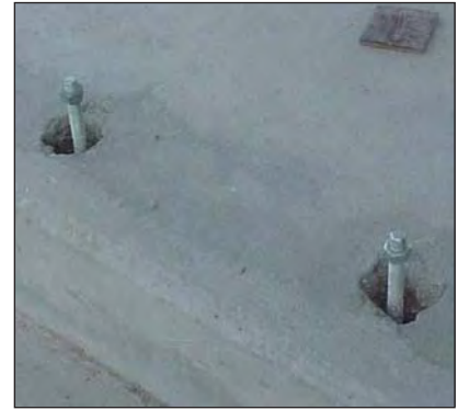
Due to site confusion, hot dip galvanized (left) and electroplated (right) holding down bolts are sometimes incorrectly mixed up.
