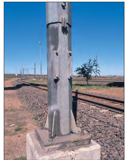
Figure 3 (top) and figure 4 (bottom). Corrosion protection of holding down bolts should be equal to that provided for main structures.
