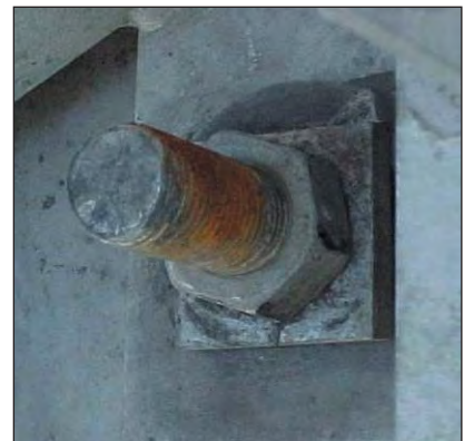
Some contractors cast-in hot dip galvanized holding down bolts and find that the supplied nuts are not oversized, resulting in the coating being removed by a tap so that the nuts may fit.
