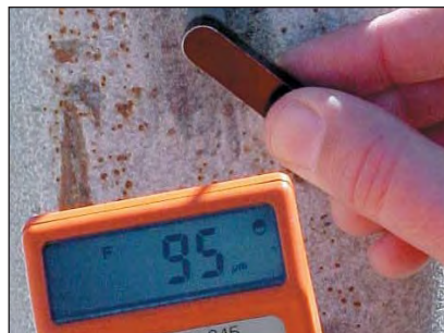
Coating thickness (95µm) on the scraped surface.
