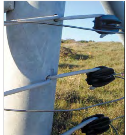
Hot dip galvanized S-Hooks are used for maintaining tension on the electrical insulators.
