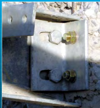
Electroplated expansion bolts offering less protection on steelwork projects that are hot dip galvanized for durability, no longer have to be tolerated by the specifiers.
