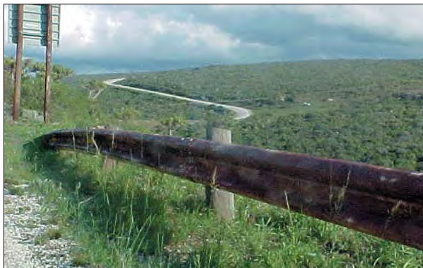
Uncoated guard rails discolour and corrode.
