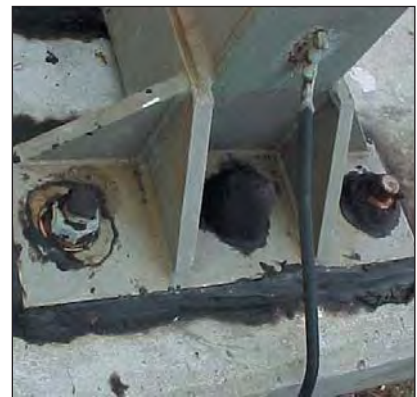
Frequently, due to last minute ordering of holding down bolts, they are installed with no coating at all and must be protected with some other method, which often requires regular maintenance.
