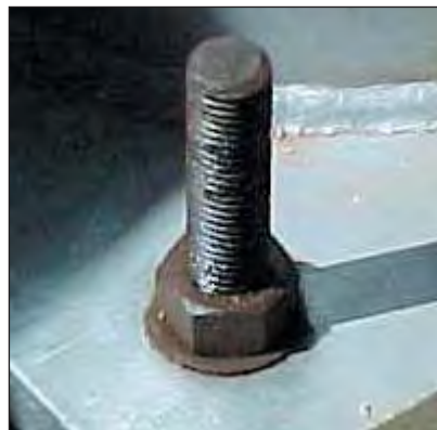
Frequently, due to last minute ordering of holding down bolts, they are installed with no coating at all and must be protected with some other method, which often requires regular maintenance.
