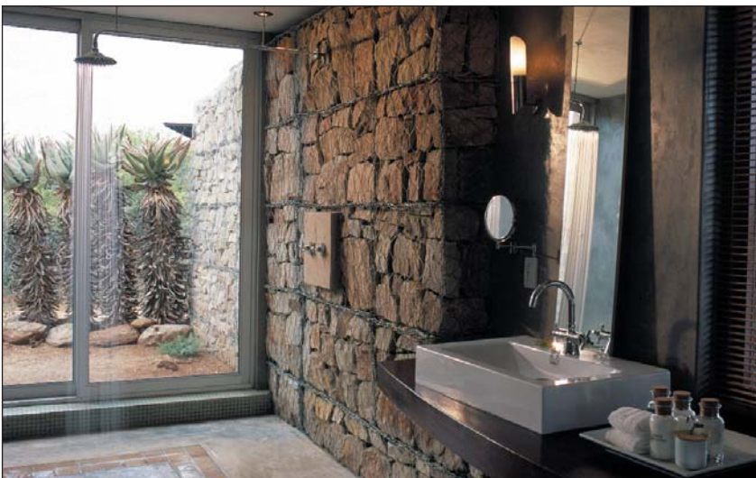
Gabion walls in the shower of one of the rooms.
