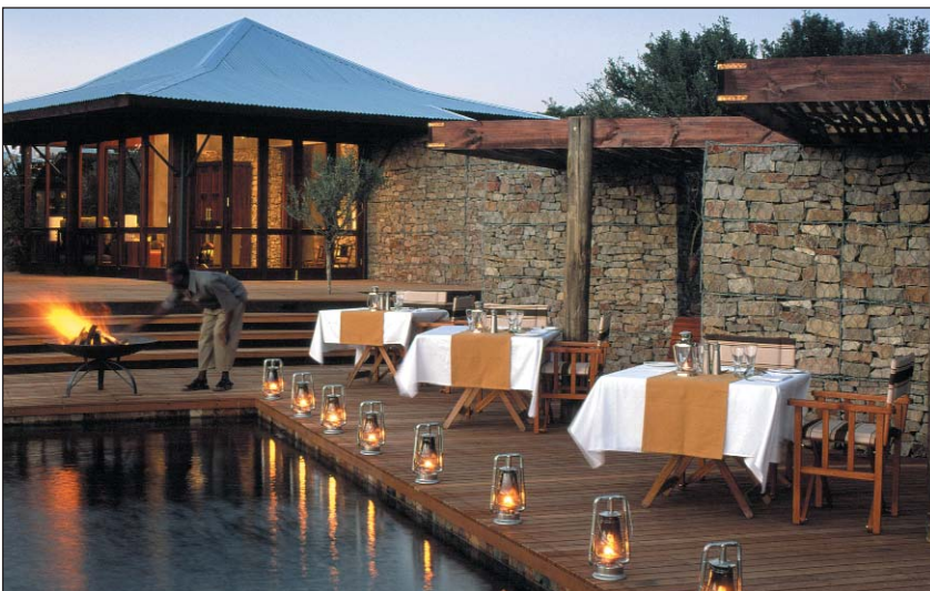
Gabion walls at the pool and dining room.
