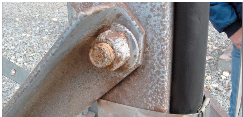
Condition of the "upper" and "lower" fastener assembly illustrating the differential rate of corrosion due to the "Time of Wetness".
