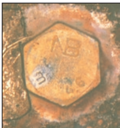
Figure 90. Galvanized bolt in contact with 3CR12 plate after 10 cycle SO 2 test. Note the cathodic protection provided by the galvanized bolt head to the surrounding steel.
