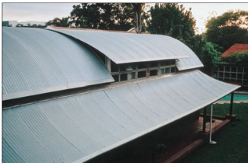
Figure 18. S-Rib galvanized steel sheeting – Z600 coating classification used for architectural applications.
