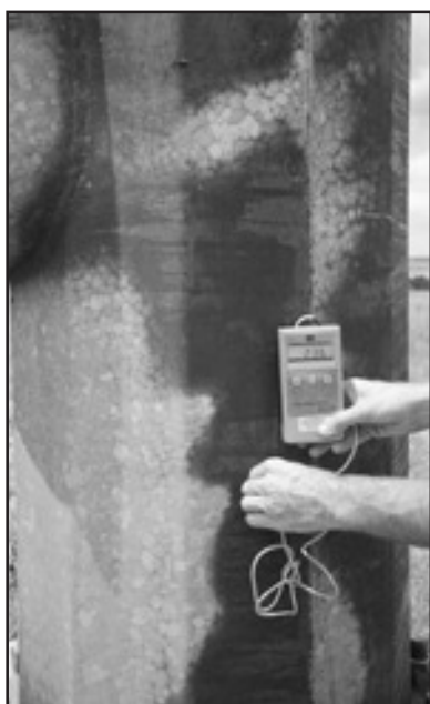
Figures 30 and 31. The galvanized coating is sometimes not uniformly grey but has a blotchy appearance with a mixture of matt, grey and shiny areas. Signs of red rust staining after several years in service is not necessarily an indication that the coating has corroded away.
