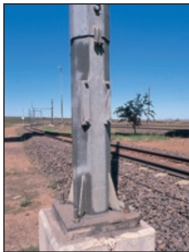
Figure 102 (left) and figure 103 (right). Corrosion protection of holding down bolts should be equal to that provided for main structures.
