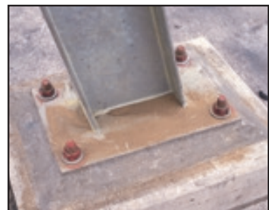
Figure 102 (left) and figure 103 (right). Corrosion protection of holding down bolts should be equal to that provided for main structures.
