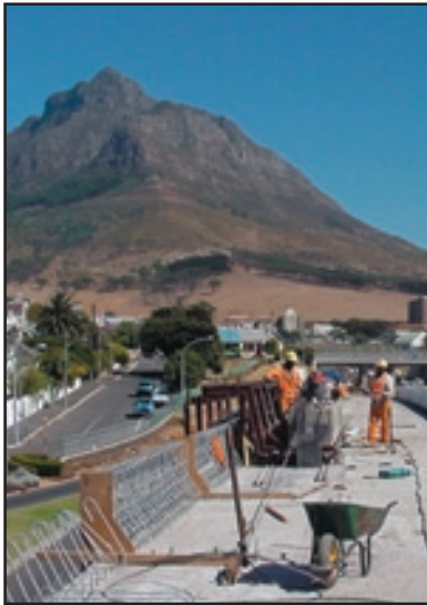
Figure 98. Hot dip galvanized reinforcing bars prior to casting concrete, marine conditions.
