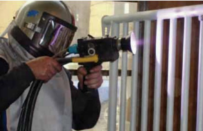
method are required. Upon contact, the particles flatten onto the surface, freeze and mechanically bond, firstly onto the roughened substrate and then onto each other as the coating thickness is increased. In thermal spraying flamespray and arcspray are normally used for finishing coatings.
