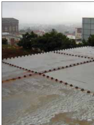
View on the roof looking north.
