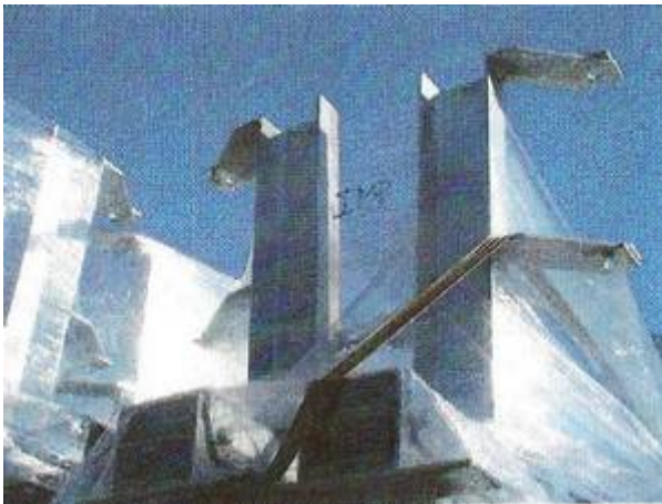
Secure and ready for the trip
